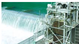
Hydro energy: hydro power plant drives
